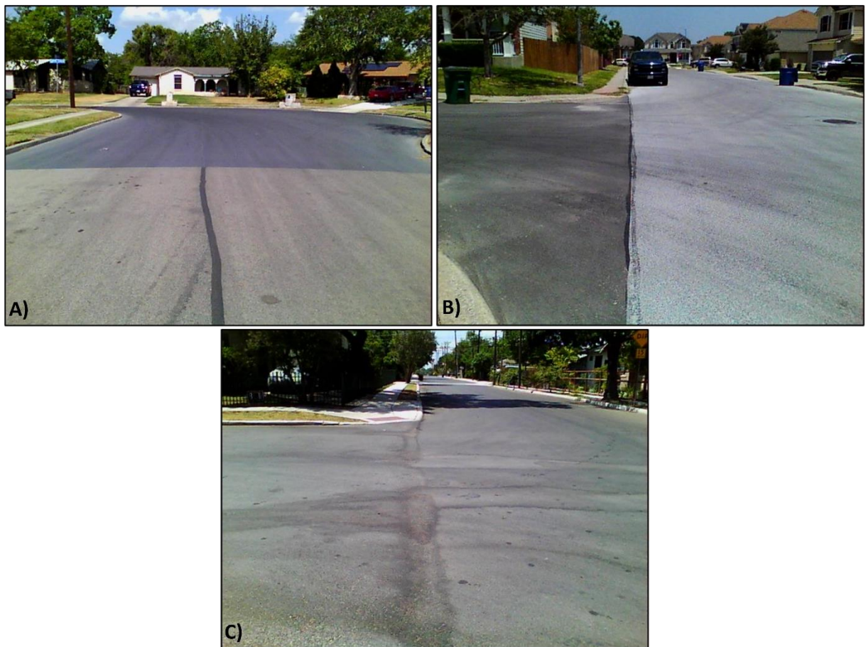
Figure 2. Examples of the cool pavement products evaluated in the study: A) Durashield at Carol Crest (cool pavement in the background with untreated road in the foreground), B) SolarPave at Mountain Star (cool pavement on the right with untreated road on the left), and C) PlusTi at Grant Avenue (cool pavement on the right with untreated road on the left).
