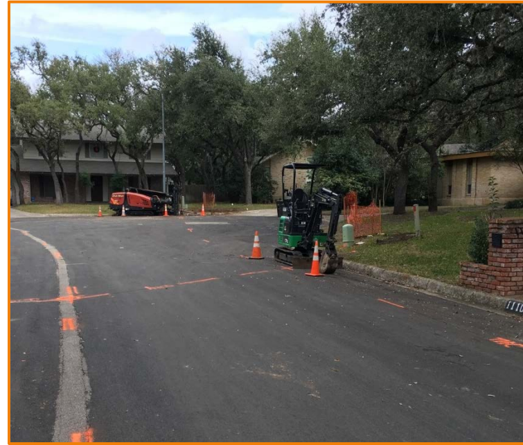
Boring & Vault Excavation
