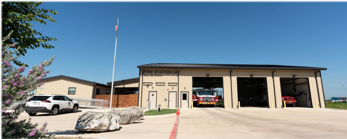
Fire Station 54 (Council District 2) Completed December 2019 2019 Temporary Capital Budget
