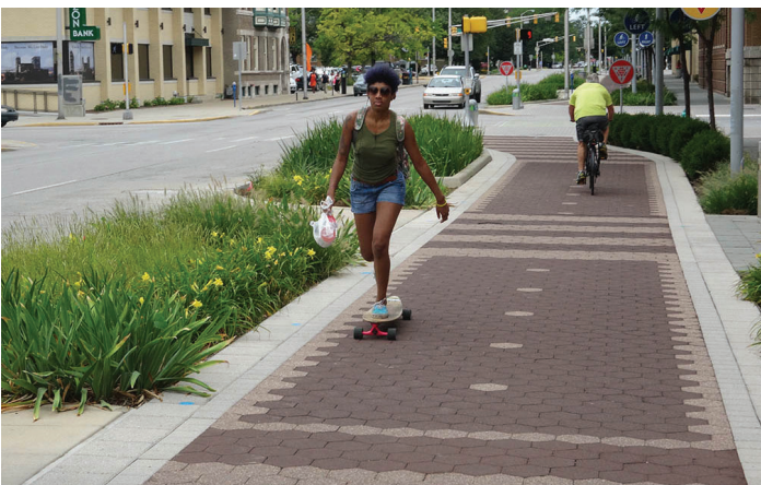
Pervious pavement (PP)
