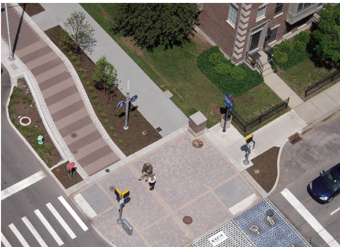
Permeable paving treatment along trail and intersection, Indianapolis Cultural Trail, Indianapolis, IN
