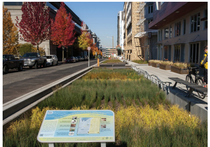
Swales in the right-of-way, Yale St., Seattle, WA
