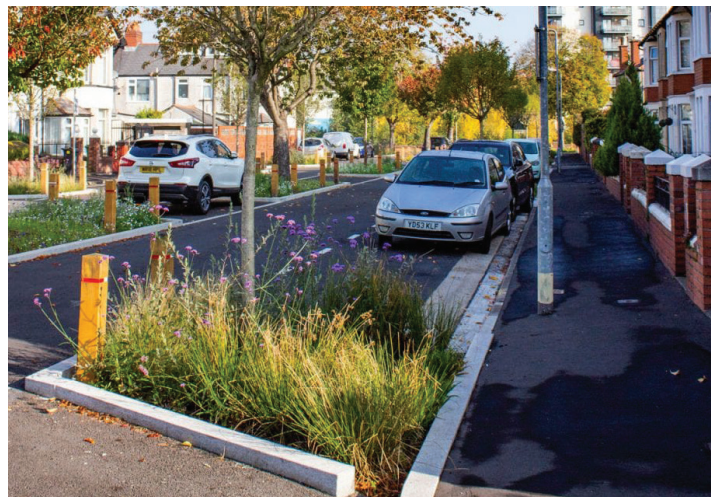
Stratacell bioretention tree planting, Greener Grange town, Wales
