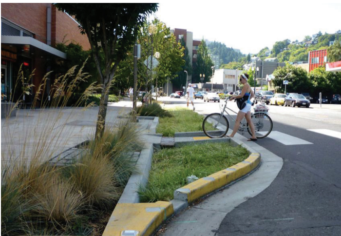
Bioretention swales; Hoboken, NJ
