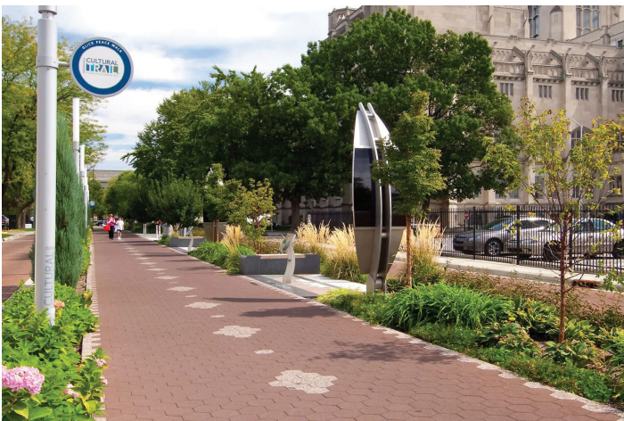
Permeable pavers, Indianapolis Cultural Trail, Indianapolis, IN
