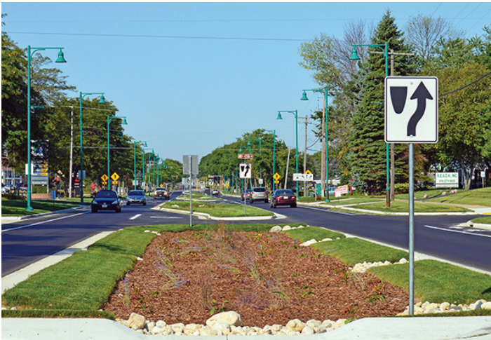
Swale in median; Bradley Road, Brown Deer, WI
