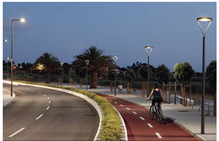
Roadway and street lamps, Rua da Pêga Redevelopment, Portugal
