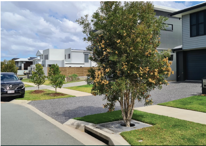
Tree wells with curb inlets in residential areas
