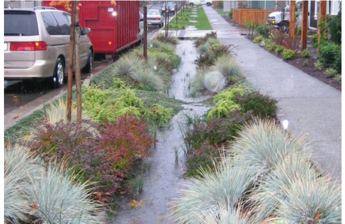
Bioretention swales (BS)
