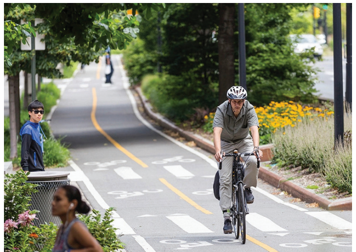
Pervious concrete treatment, Queensboro Bridge Greenway, NY
