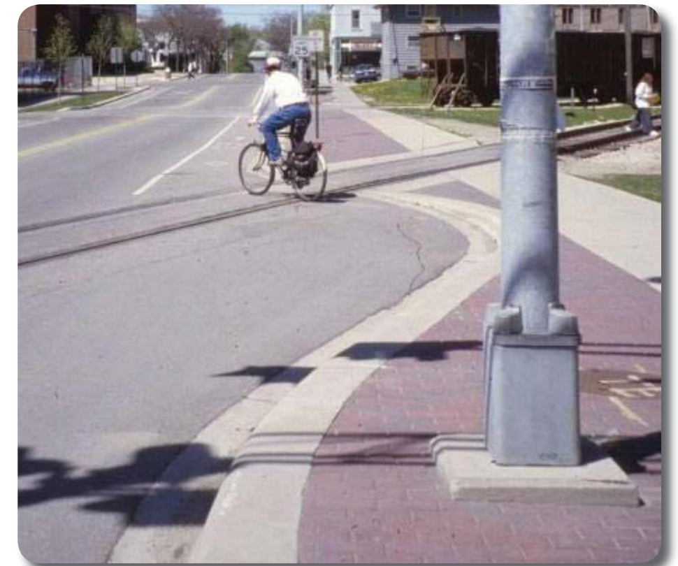
The recommended design treatment at diagonal railroad crossings. Image Source: Toole Design Group
