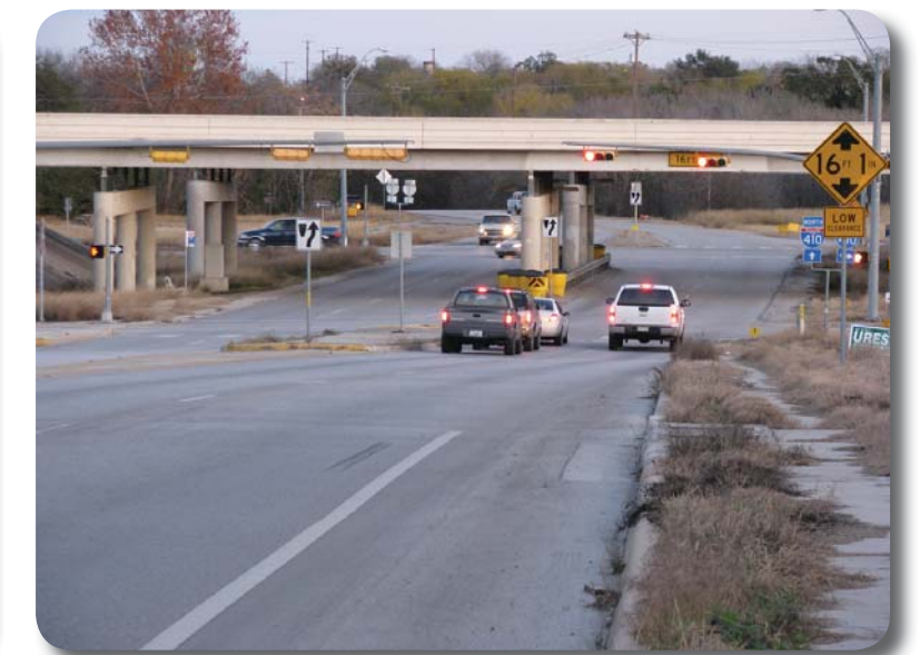
A shoulder disappears as it approaches a bridge, which imposes a barrier. Image Source: Halff Associates, Inc.
