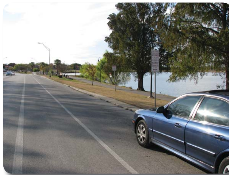
A bike lane on Woodlawn Ave connects to Woodlawn Park. Image Source: Halff Associates, Inc.
