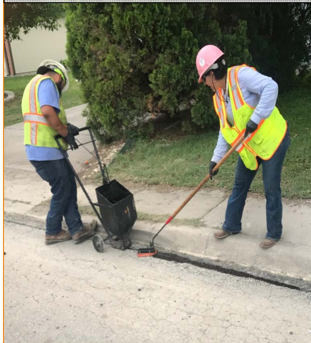
Sealant installation
