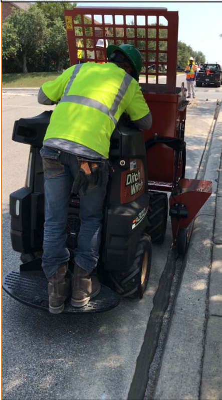
Pilot #2: CLSM backfill
