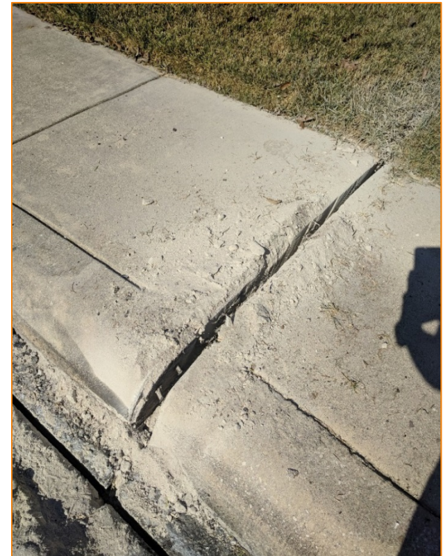
Curb & sidewalk cuts
