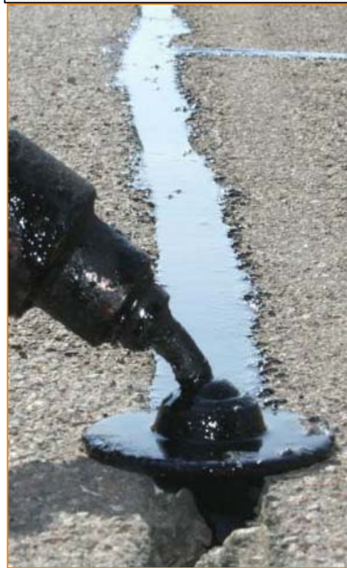
Pilot #3: Sealant application
