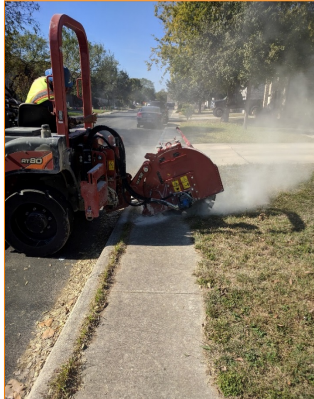
Curb & sidewalk cuts
