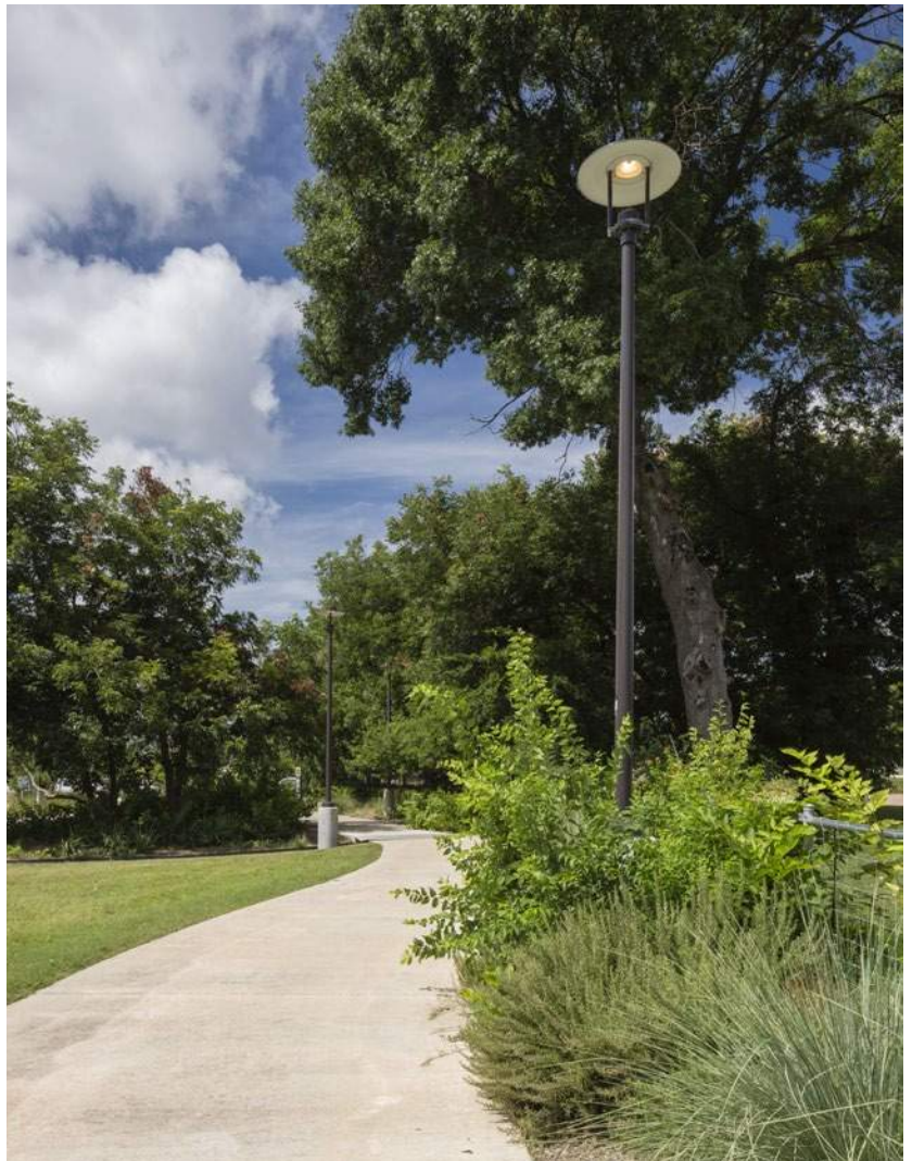
Figure 3.16a: Local example of full-cutoff, DarkSky Approved certified fixture
