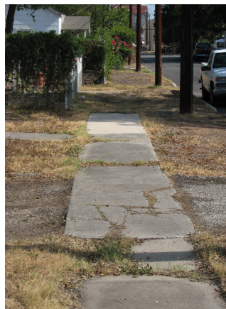
Broken sidewalks along Mesquite that need to be replaced.
