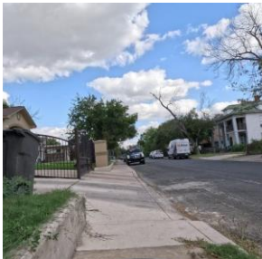
Excessive Cross Slope
