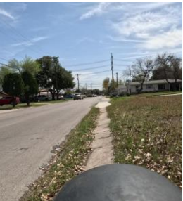
Excessive Cross Slope
