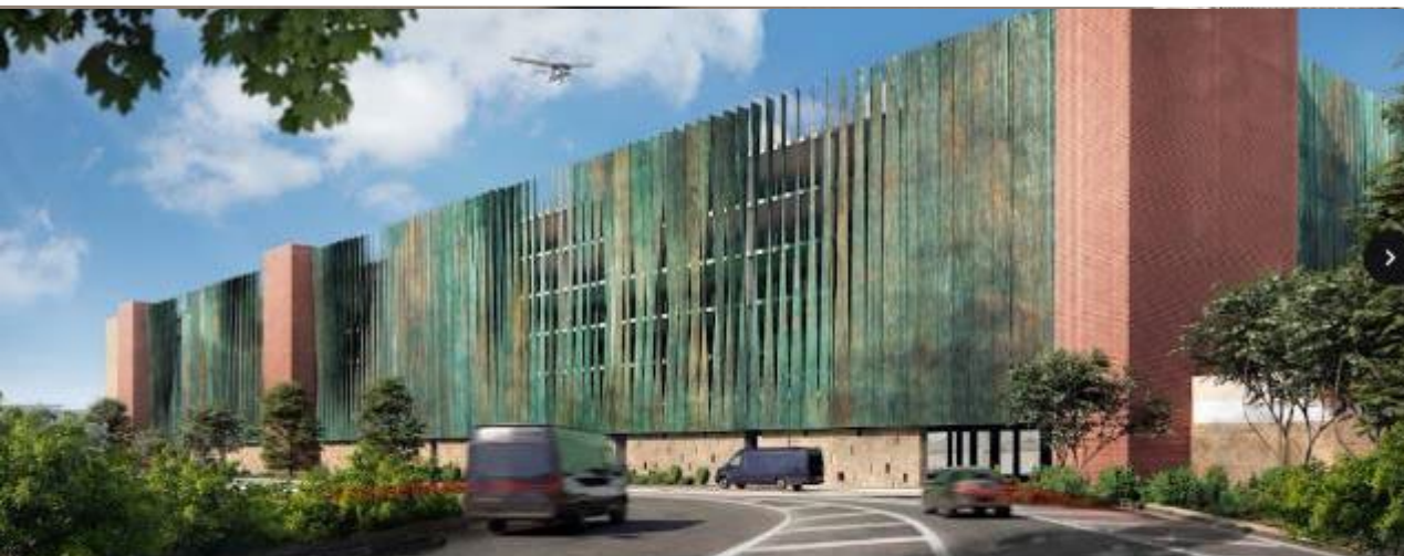
Terminal C Parking Structure & Ground Transportation Center
