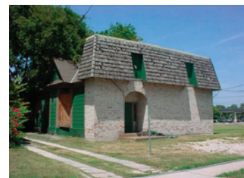
Appropriate design guidelines can assist property owners in making appropriate decisions regarding alterations and additions.
