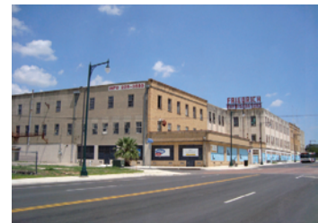
East Side- Friedrich Refrigeration
