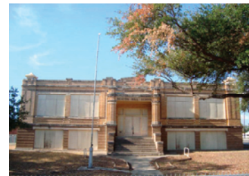
Historic preservation should be considered in all planning processes conducted by municipal departments and affiliated agencies
