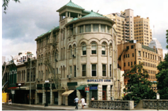
Clifford Building, H.H. Hugman, Alamo Plaza Historic District
