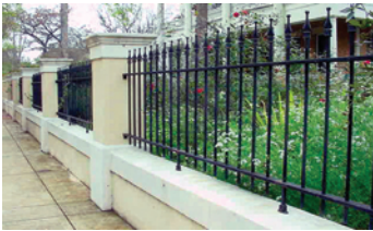
Historic fencing and other landscaping features should be documented during surveying activities.
