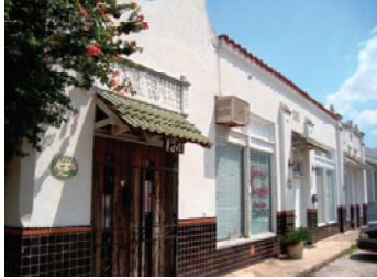
Neighborhood commercial building in Lavaca.
