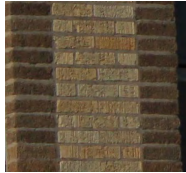
Striated Wire Brick Veneer
