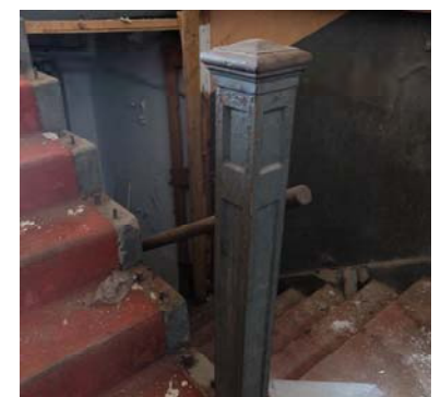
Original cast-iron balustrade
