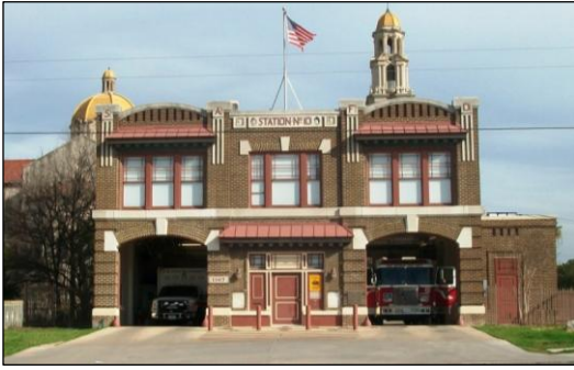
Fire Station No. 10 1107 (1103) Culebra
