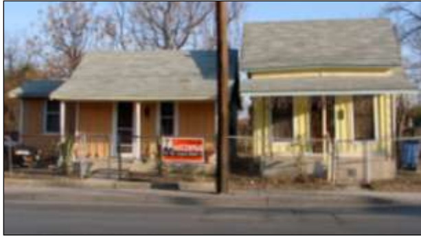
Shotgun Houses 1107 Guadalupe Street
