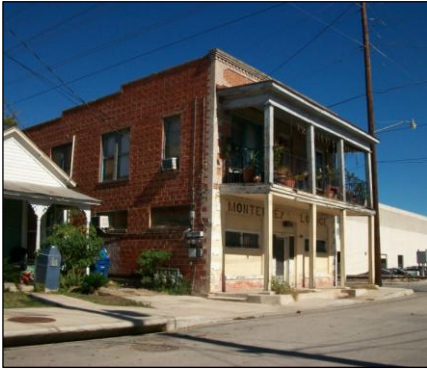
Building 1001 N. San Marcos (401 Arbor Place)
