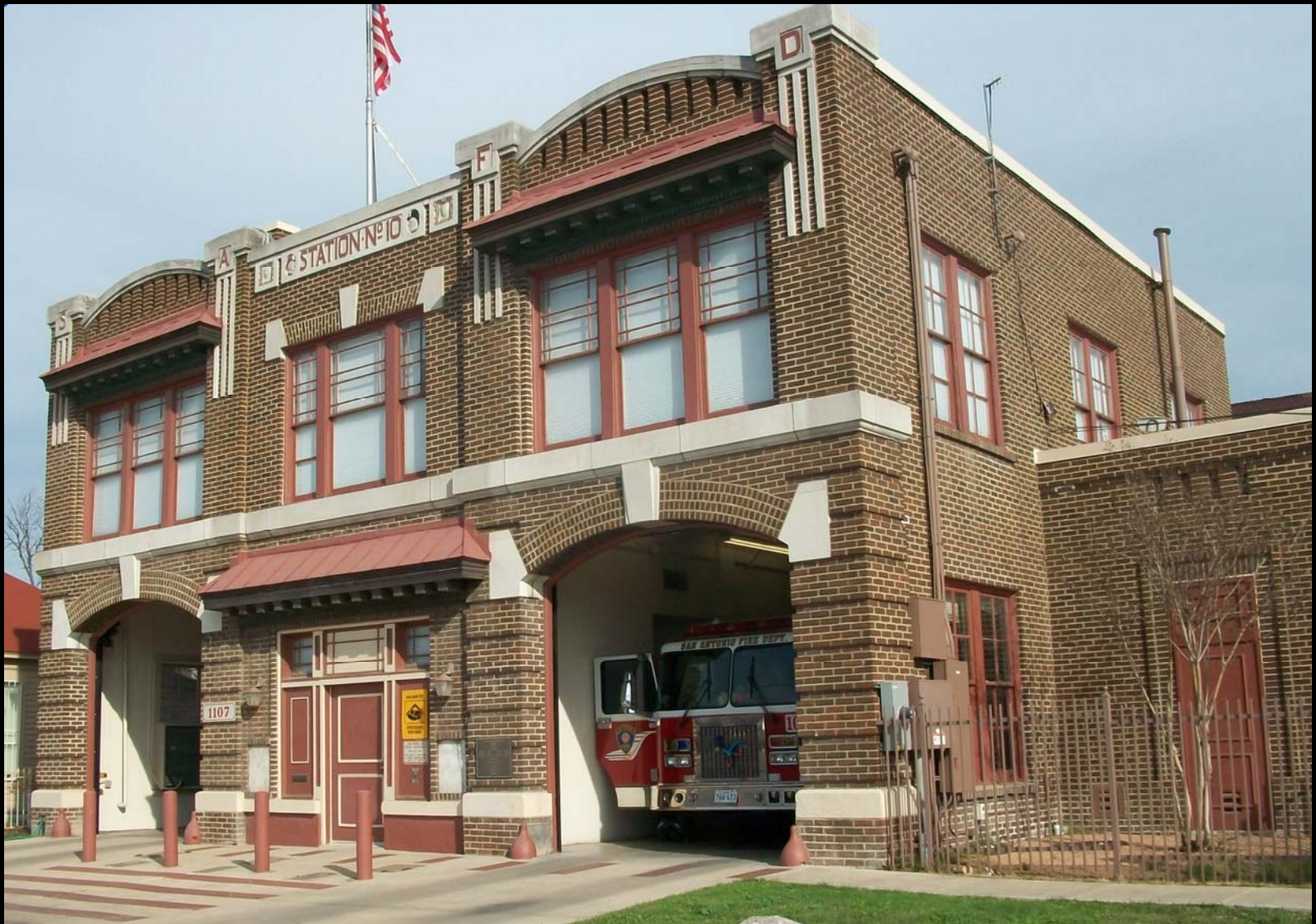
Fire Station No. 10 1107 Culebra
