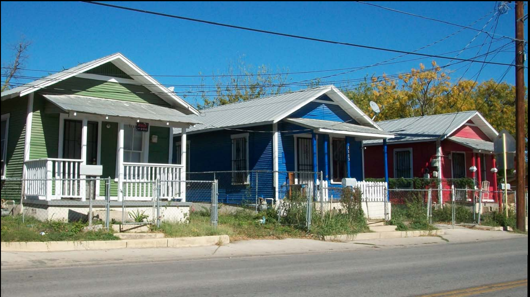
Shotgun Houses 1113 Guadalupe Street
