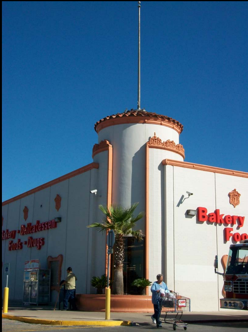
Former Joske's at Las Palmas 803 Castroville Road
