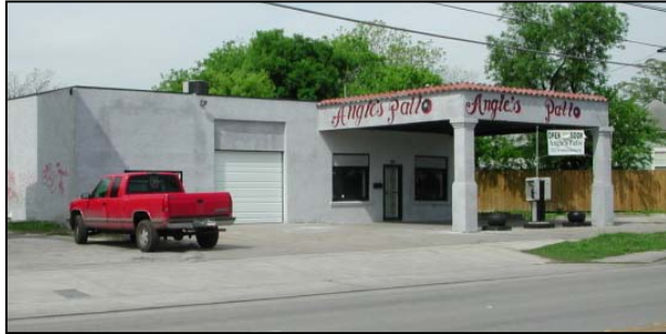
Former Gas Station 323 Fredericksburg Road
