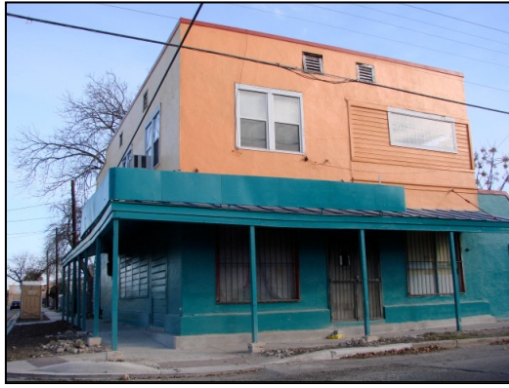
Commercial Building 1425 El Paso
