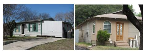
Incompatible building materials used in renovations and additions can alter the integrity and character of the structure.
