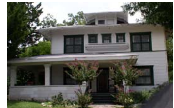
Typical two-and-a-half story residential structure
