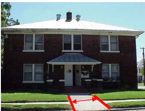
Typical example of front walkway on a residential property; Multi-family structures require a 4 foot walkway
