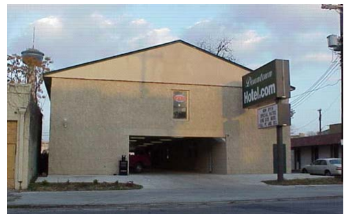
Example of inappropriate entrance configurations in a commercial area
