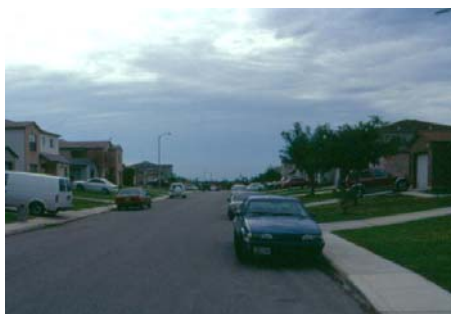
Non-conforming driveway and sidewalk configuration
