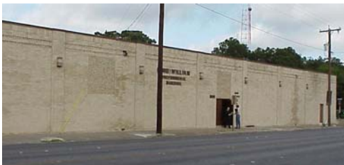
Non-conforming example of a commercial building with no window openings
