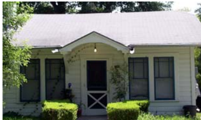
Appropriate wood window screens
