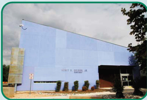
GUERRA LIBRARY LIGHTING RETROFIT $150,000
