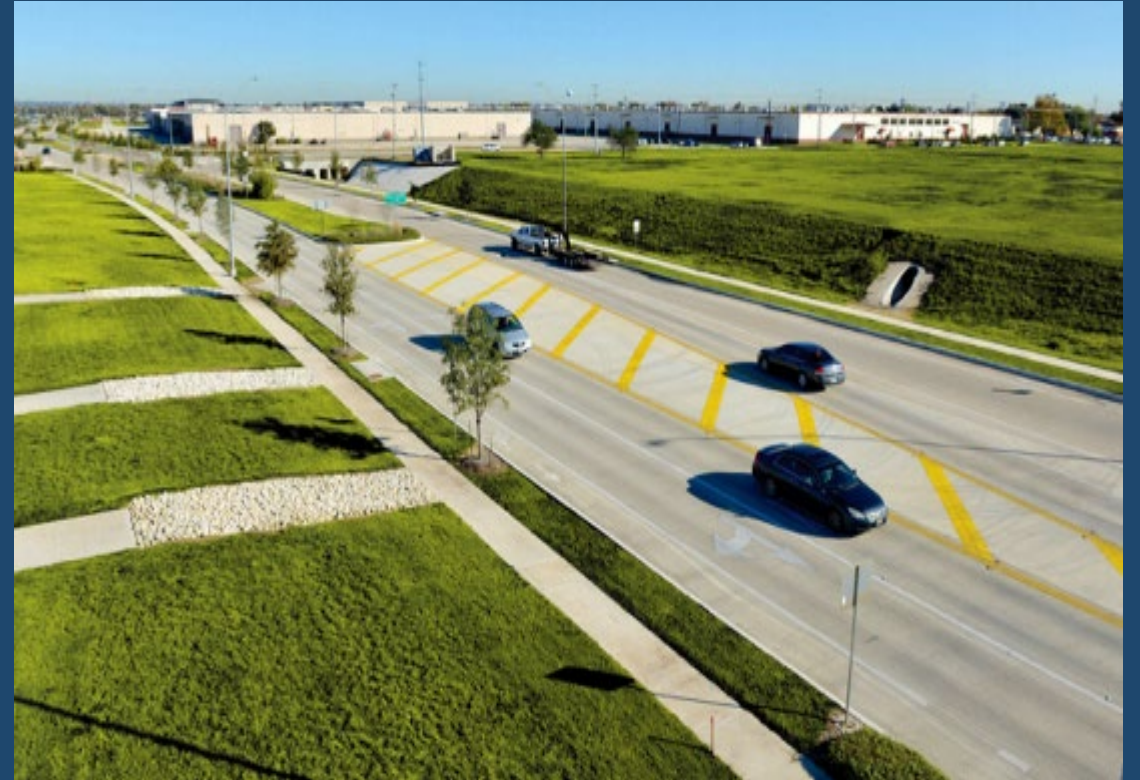
Port San Antonio (Comprehensive Drainage Improvements)
