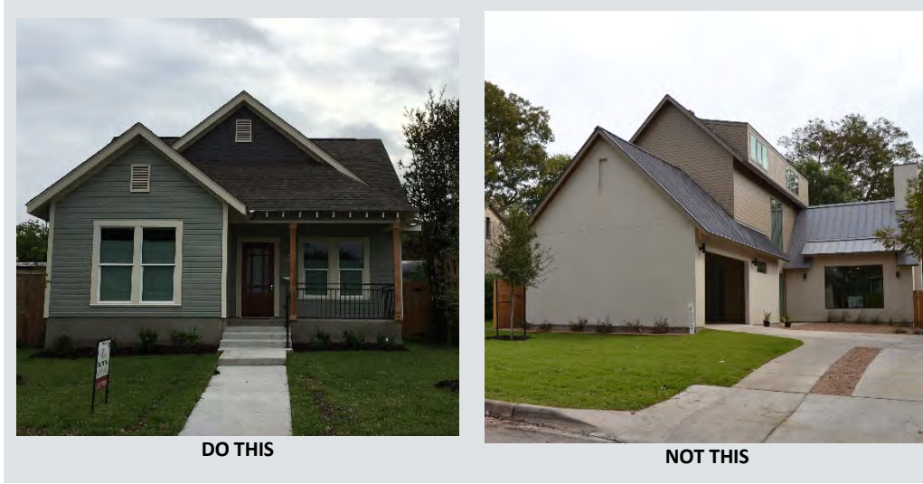
Figure 6.3.1. Examples of two new infill houses in a historic neighborhood – one using an appropriately oriented front door facing the street (left), while the other uses an inappropriate front door hidden from the front façade (right). Source: Photos by the COSA OHP and HHM, 2021.
