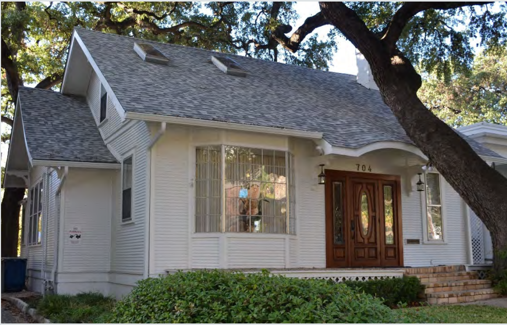
Figure 4.4.1. Example of an inappropriate alteration that changed the size and shape of an original window opening. Source: Photo by HHM, 2019.
