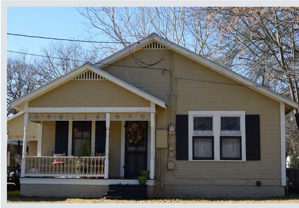
Figure 4.6.2. Example of a porch with a non-original Victorian-inspired “gingerbread” frieze and turned posts and balusters that do not match the period or original style of the house. These elements create a false historic appearance. Removal of the brackets is recommended but not required. Source: Photo by HHM, 2020.
