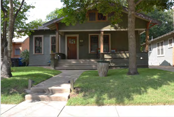
Figure 2.2.19. Example of a sidewalk and walkway in the River Road Historic District, with steps to navigate the change in grade between the street and the lawn. Source: Photo by HHM, 2021.
