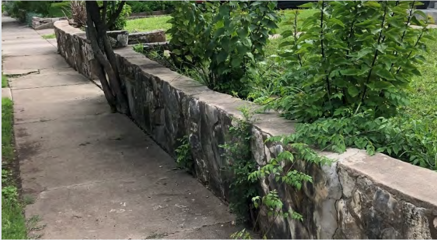
Figure 2.2.14. Example of a retaining wall in the River Road Historic District. Source: Photo by HHM, 2021.
