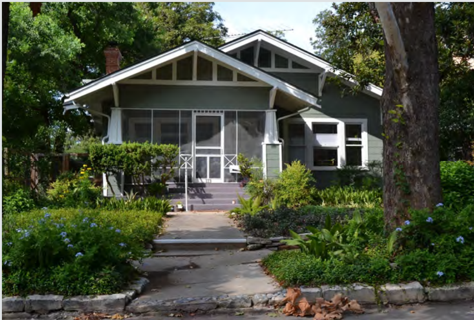
Figure 4.6.1. An example of a simple, transparent screened enclosure on a historic front porch that allows visibility of the character-defining features of the historic Craftsman house. Source: Photo by HHM, 2021.
