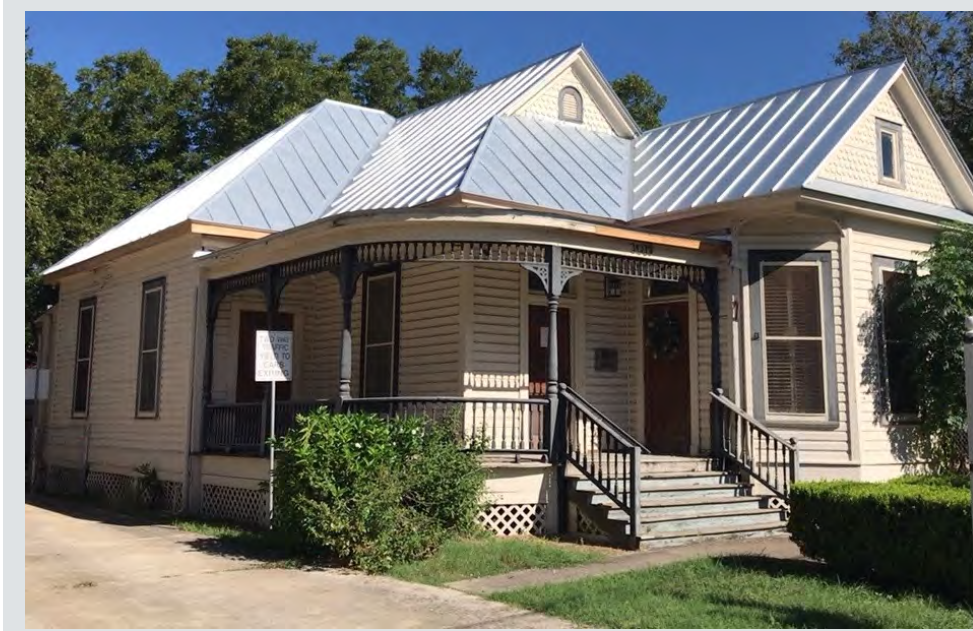
Figure 4.5.2. Example of a metal roof on a historic bungalow. Metal roofing is only appropriate throughout the district, provided that its installation does not remove or damage character-defining historic features. For buildings dating before 1945—like this one—the ridge cap and seams for the metal roof are recommended to comply with the “Checklist for Metal Roofs” in the citywide guidelines. Source: Photo by OHP, 2022.
