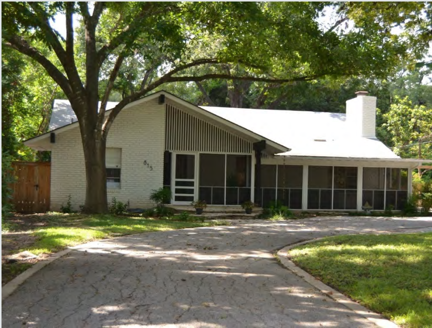
Figure 2.1.12. Example of a Ranch style house in the River Road Historic District. Character-defining features found on this selected example include:
