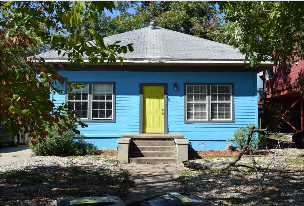
Figure 4.4.2. Example of windows on the primary façade of a historic building that are both non-original and non-compatible. Although these windows likely are more than 25 years old, they do not need to be preserved since they are non-compatible. If the owner chooses to replace these windows, the new windows that are visible from the public right-of-way must be similar to those found on other buildings from the same period in the district. Aluminum windows would be allowable provided all other guidelines for windows can be met (dimension, profile, operation, etc.) Proactive replacement of the windows is encouraged but not required. Source: Photo by HHM, 2019.
