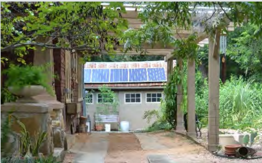
Figure 4.8.1. Example of a solar panel on a roof of a detached garage. Source: Photo by HHM, 2021.
