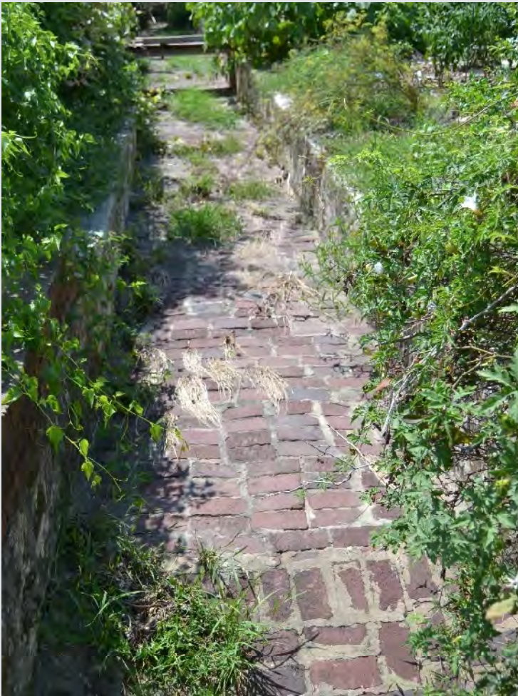
Figure 2.2.2. Section of a canal comprising part of the acequia in the River Road Historic District. Source: Photo by HHM, 2021.
