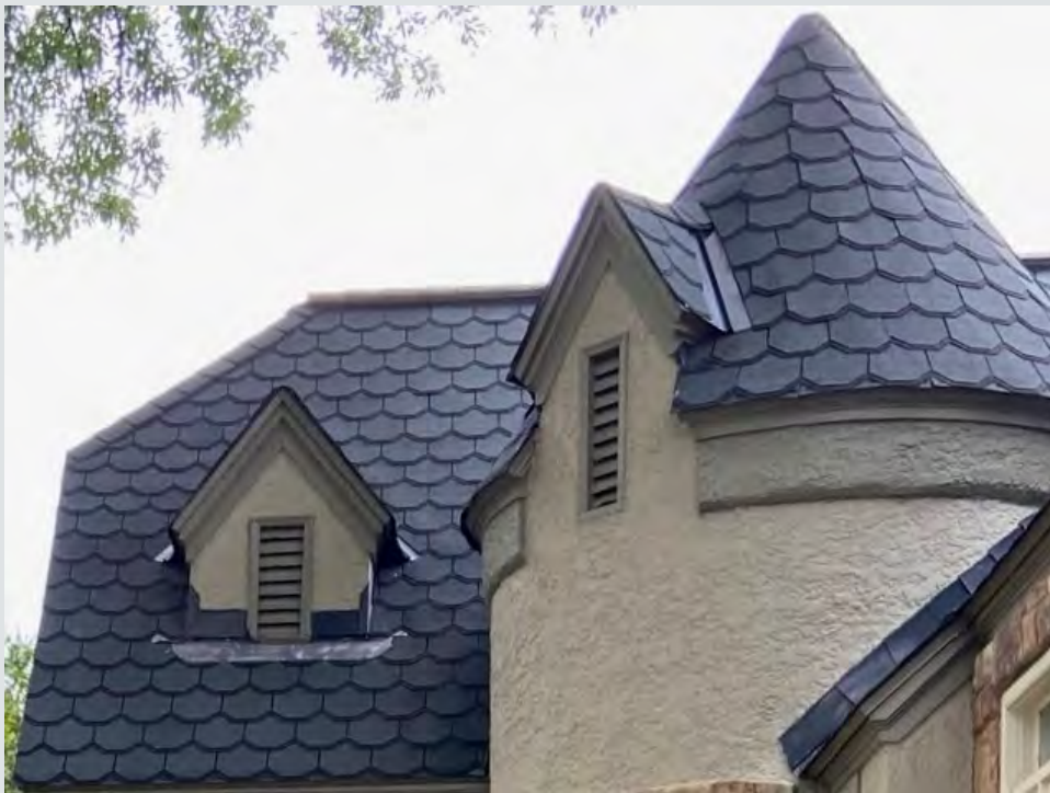
Figure 4.5.1. Example of a new roofing material that makes an effort to be consistent with the building’s style. This roof replaced a conventional rectangular-composite shingle roof (visible in Google Street View photos from 2007), so no historic materials were removed or damaged for the installation of this roof. Source: Photo by HHM, 2021.
