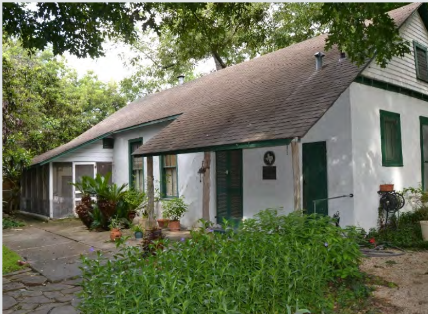
Figure 2.1.2. Example of the Spanish Colonial style house (Zambrano House) in the River Road Historic District. ii Note that this example uses rammed earth construction. Character-defining features found on this selected example include:
