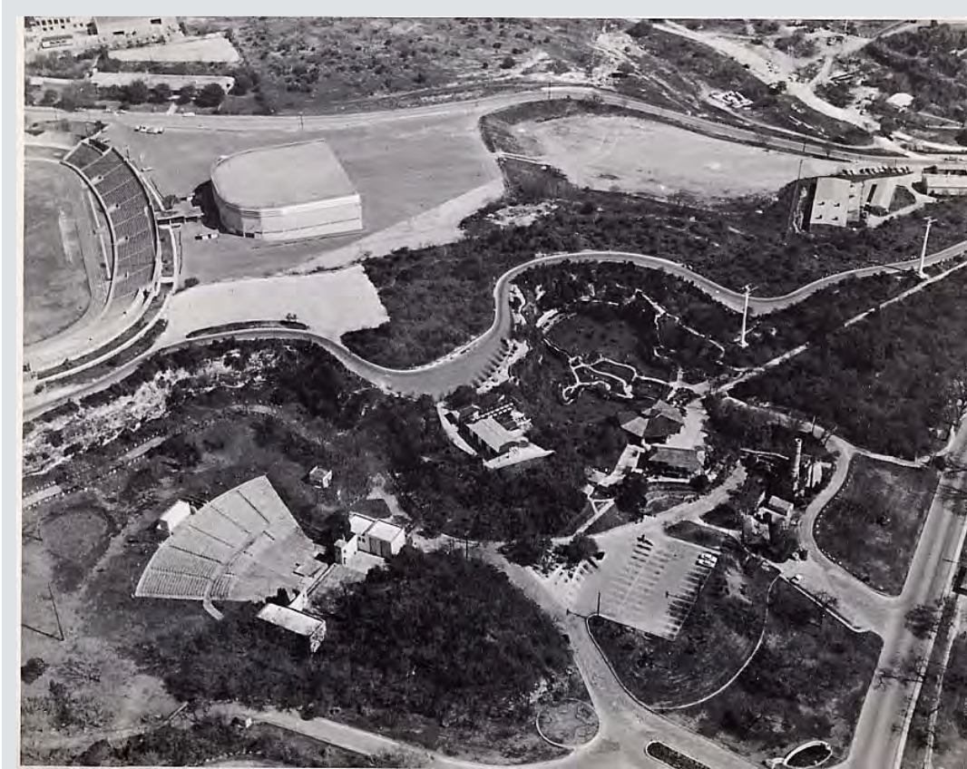
Figure A.14. Aerial view of U.S. 281 right-of-way between Alamo Stadium and the Sunken Garden Theater. Courtesy: Texas Department of Transportation.
