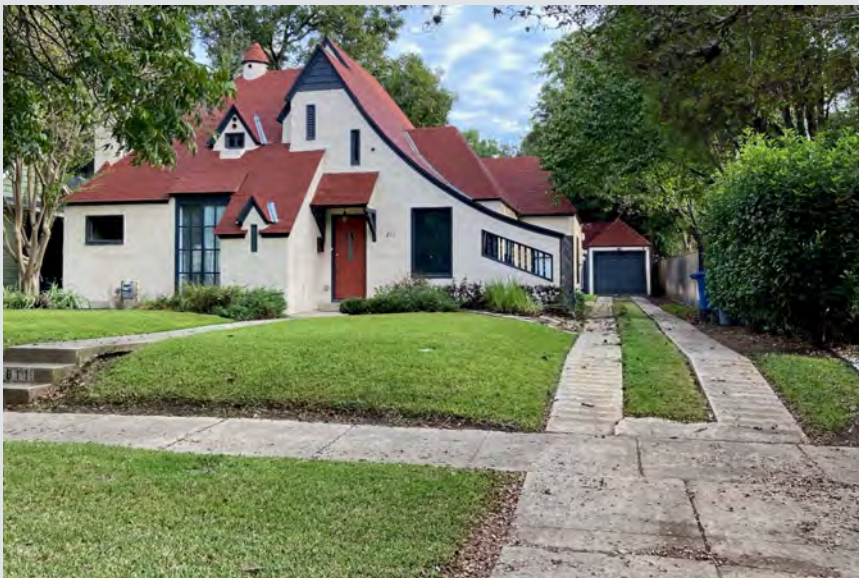
Figure 2.2.15. Example of a concrete ribbon driveway in the River Road Historic District. Source: Photo by HHM, 2021.
