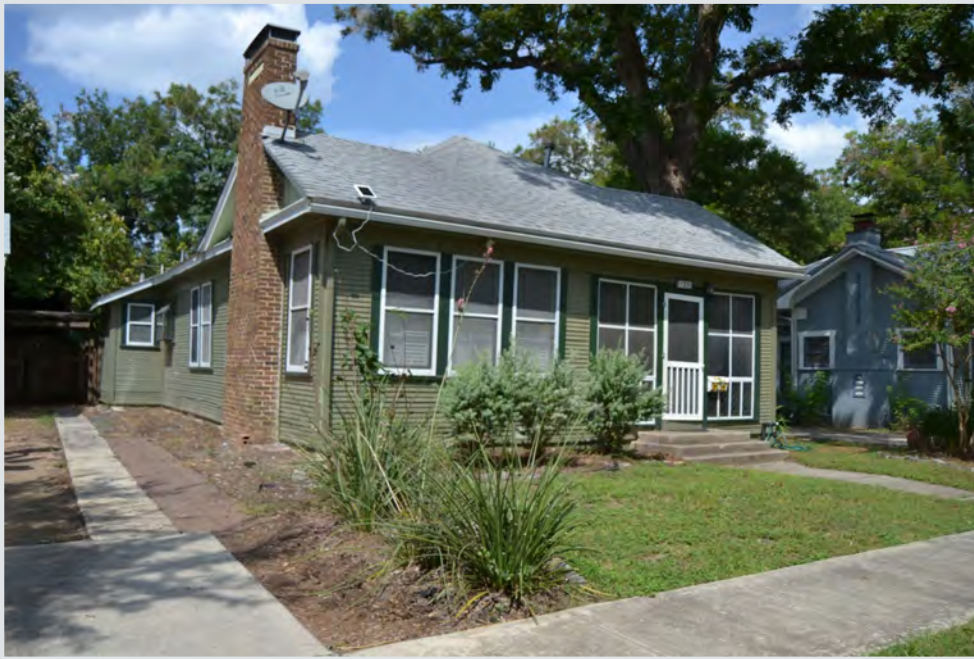
Figure 4.4.3. Example of compatible window screens that use a minimal profile and non-reflective screening so that they do not damage or obscure historic window features. Source: Photo by HHM, 2021.
