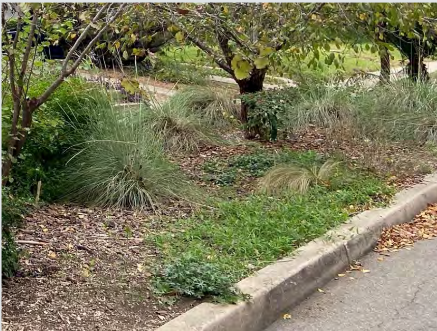
Figure 2.2.17. Detail of a historic curb profile in the River Road Historic District. Source: Photo by RRNA, 2021.
