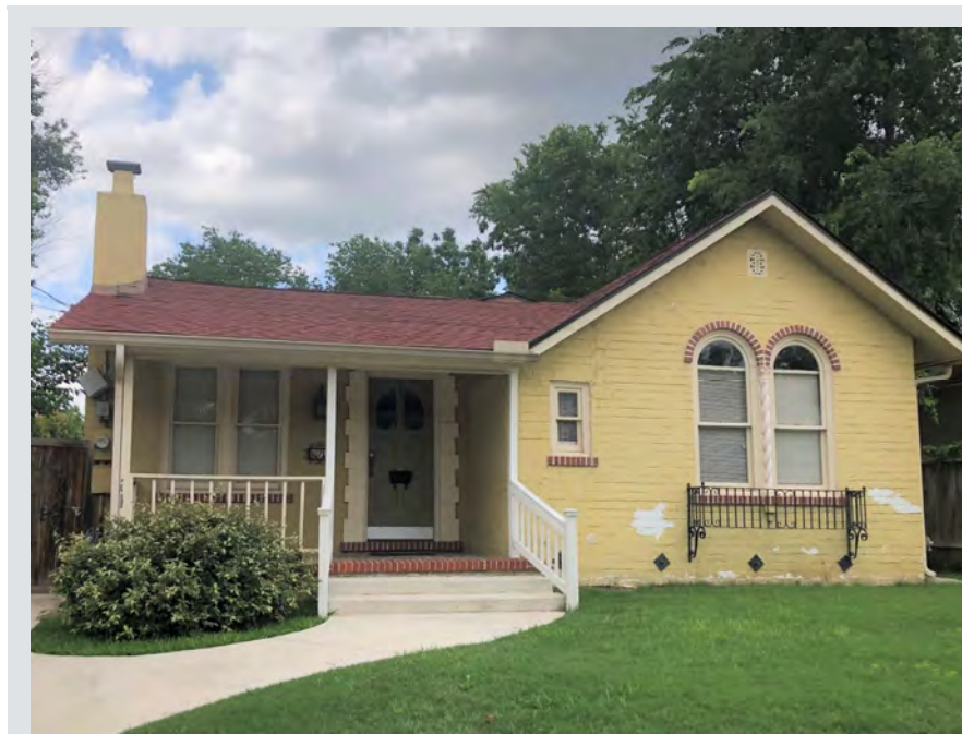
Figure 4.3.1. Example of a preserved historic door and door surround that are character-defining features of this house. Source: Photo by HHM, 2021.
