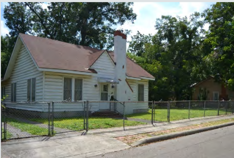
Figure 2.2.11. Example of a historic-age chain-link fence surrounding the front and backyards of a property in the River Road Historic District. Source: Photo by HHM, 2021.
