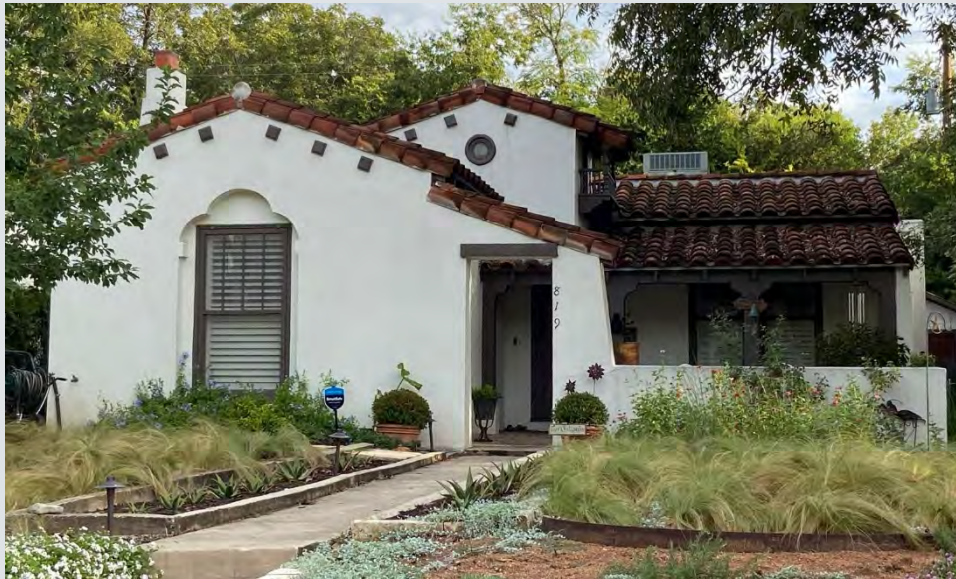
Figure 4.2.3. Example of a house preserving the original stucco exterior and terra-cotta roof tiles. Keeping the original texture of the stucco exterior is important to preserve this architectural style, as is preservation of the character-defining historic roof tiles. Source: Photo by HHM, 2021.
