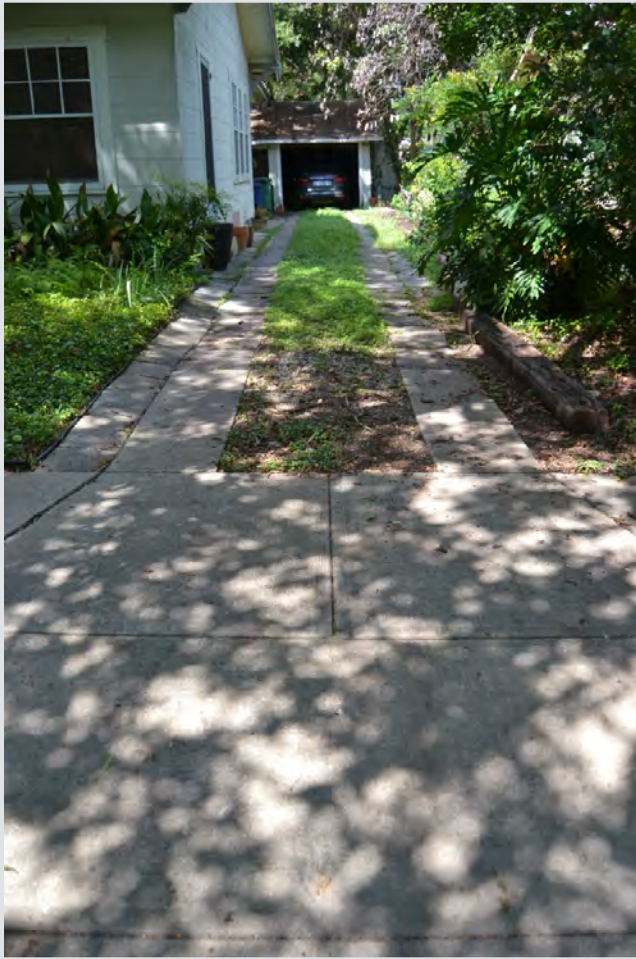
Figure 4.7.1. Example of an original ribbon driveway in the River Road Historic District. Source: Photo by HHM, 2021.
